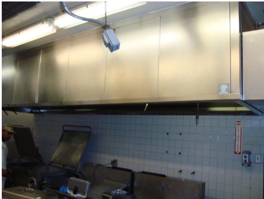
Figure B-2. Kitchen hood that is good candidate for variable air flow.
