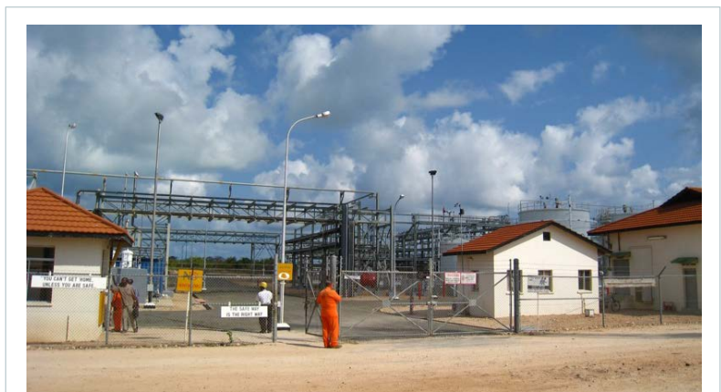
Songo Songo gas power plant in Tanzania.
